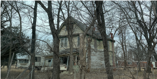
▲ Figure B.6: Single-Family Home in Dilapidated Condition
