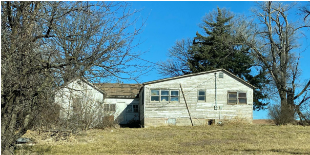
▲ Figure B.5: Single-Family Home Needing Substantial Rehabilitation
