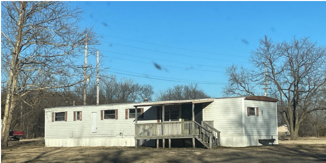
▲ Figure B.2: Mobile Home in Sound Condition
