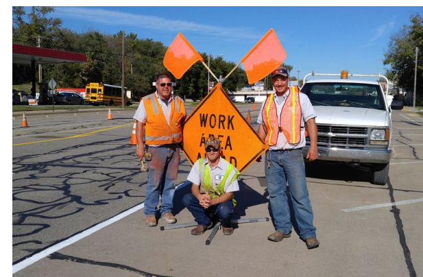
Figure 17: City Crews Striping the Roadway
