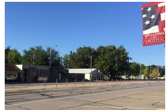
Figure 21: Center Median Pylons
