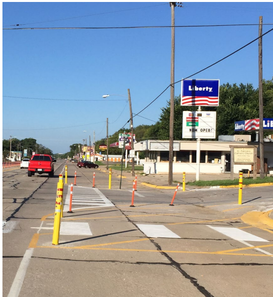
Figure 22: Semi-Permanent Curb Extensions
